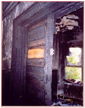
SECOND is the width of the pocket door wall. This is a much wider wall that is not only designed to house a sliding pocket door, but is also a large opening into the buildings structure. This opening could easily allow fire to gain access to the building's void spaces.
